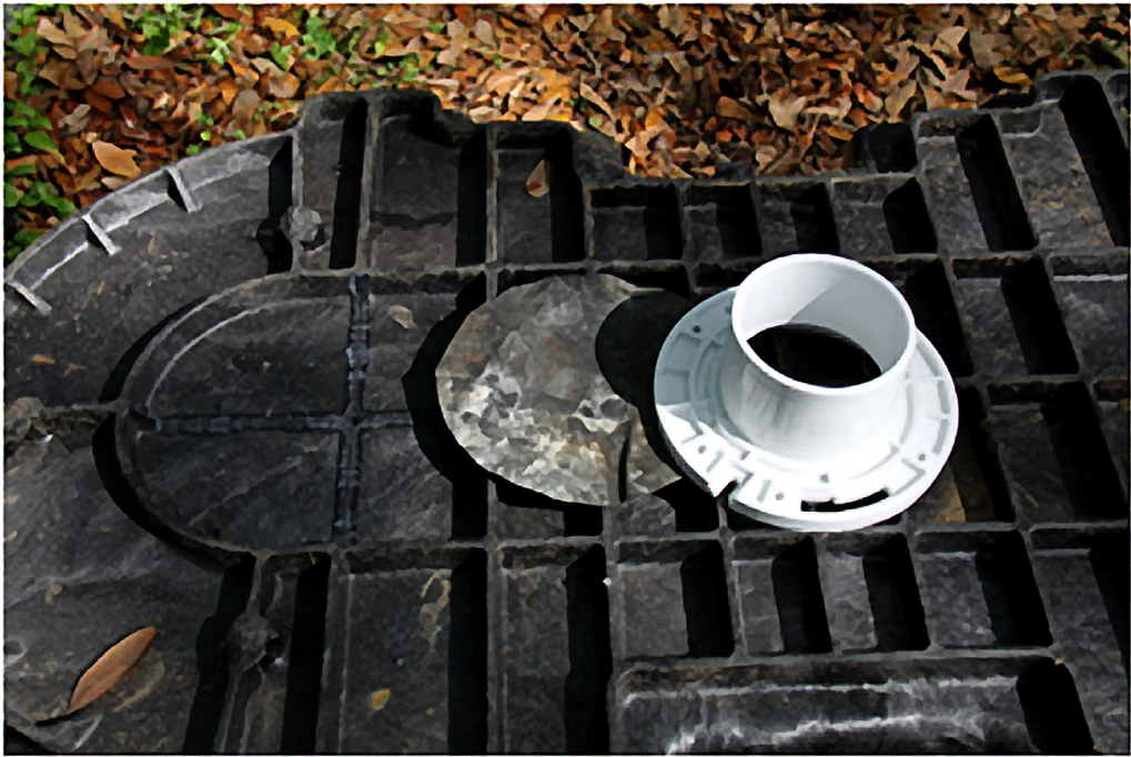
Photo 5: Preparing to install sludge drain.
